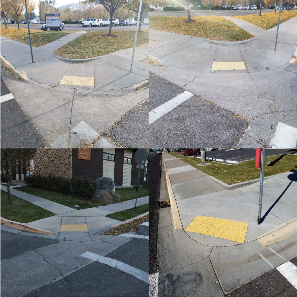
Figure 8 Examples of Combination Curb Ramps
