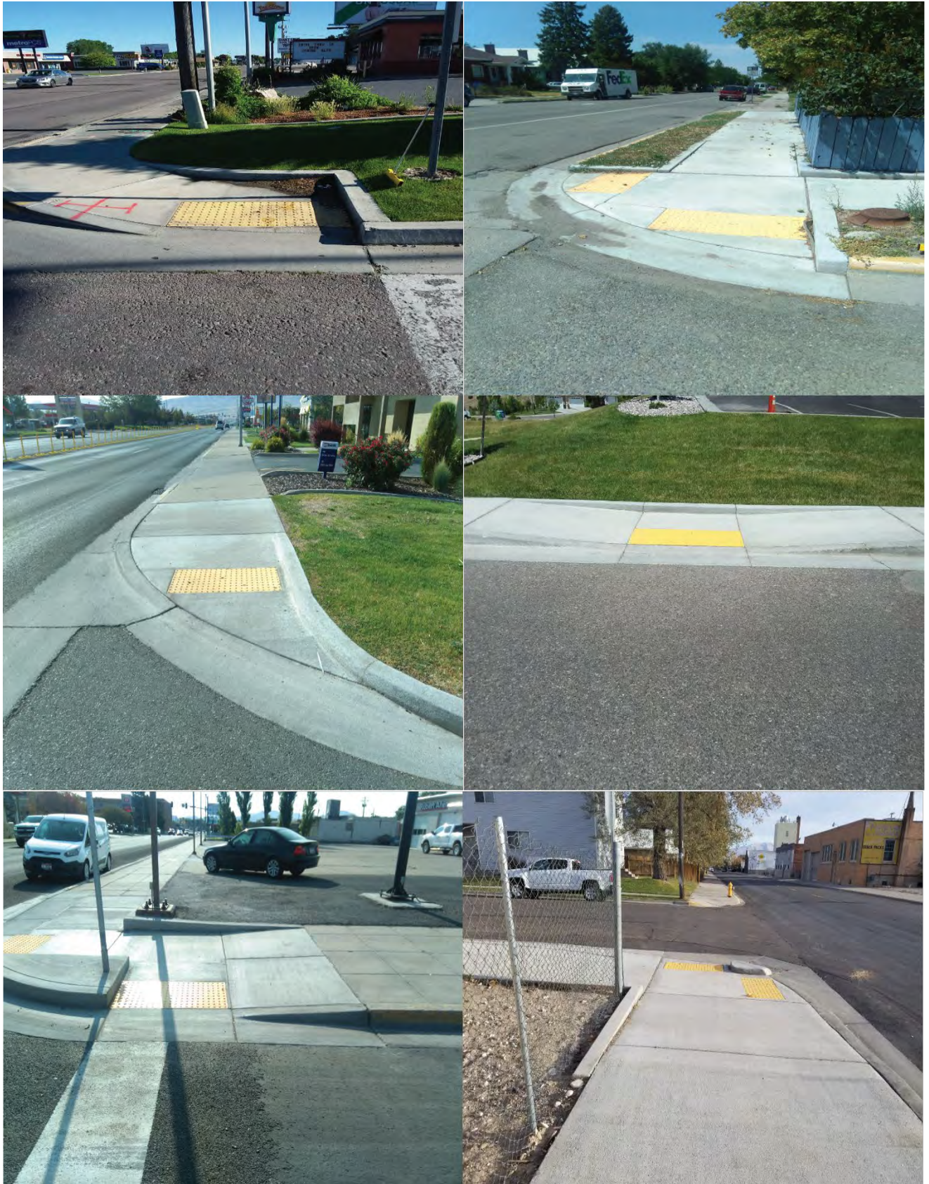
Figure 3 Example of Parallel Curb Ramps
