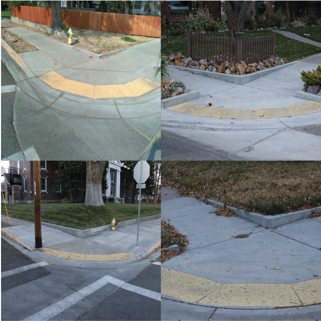
Figure 7 Examples of Blended Curb Ramps
